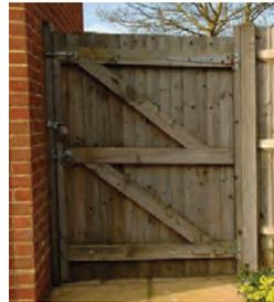
Gates should be secured using a quality, close-shackle padlock or fitted with a shroud to prevent leverage to a standard padlock.
